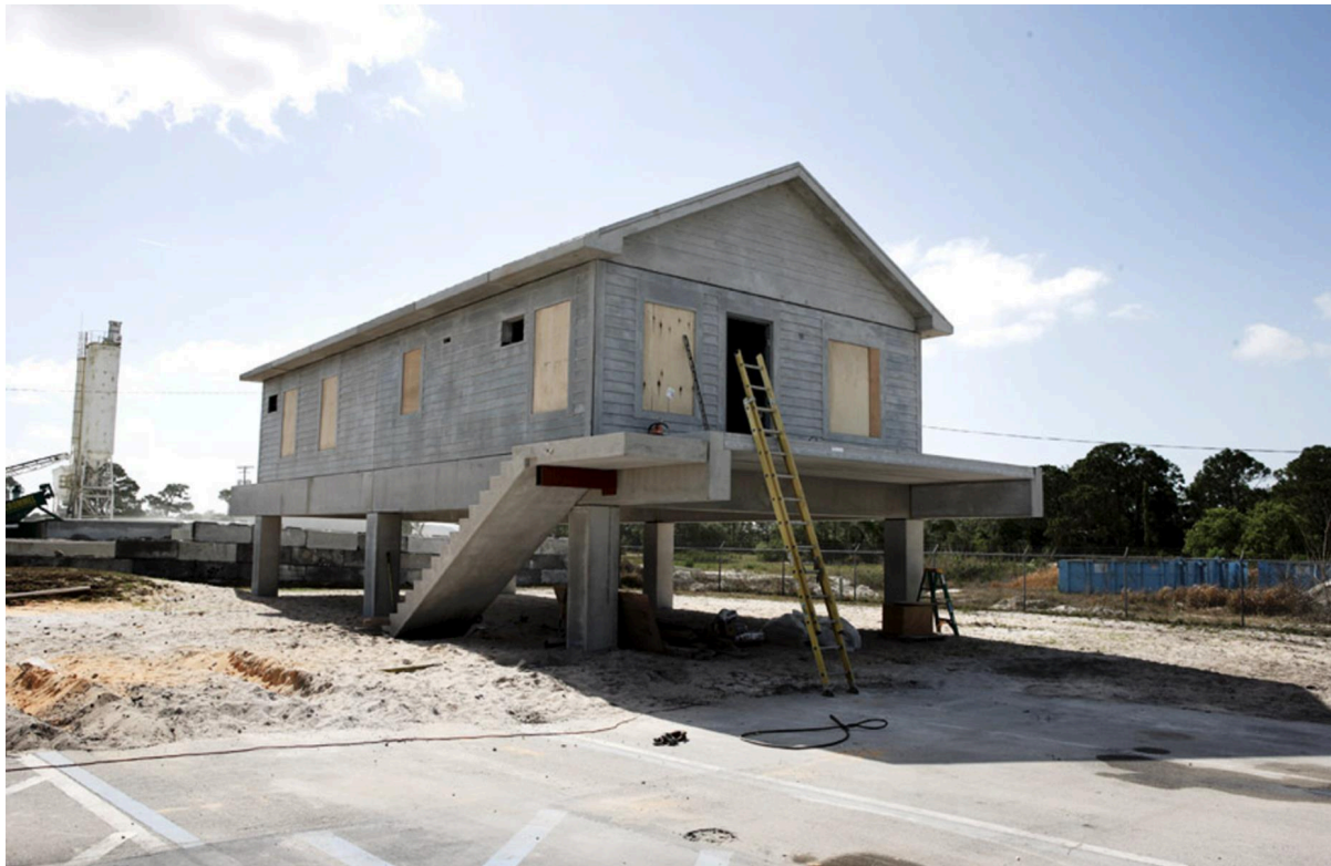
Figure 5: Elevated home that utilizes concrete in foundation and staircase [14].
