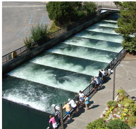
Fig. 2: A fish ladder constructed at Bonneville Dam in Oregon (Graham, 2006).
